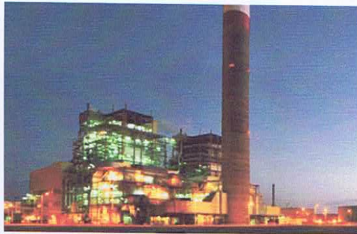
Sidi Krir power plant
